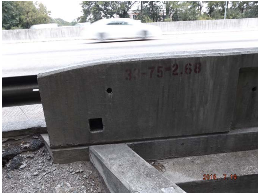
BRIDGE # - BRIDGE RAIL - RIGHT - SPAN 1
