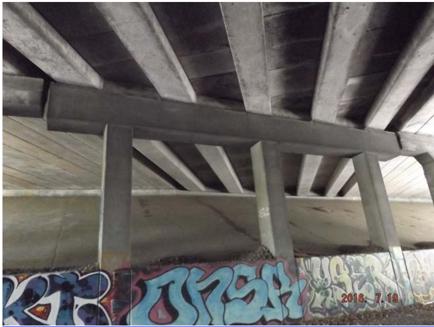
SUPER/SUB STRUCTURE - CENTER
